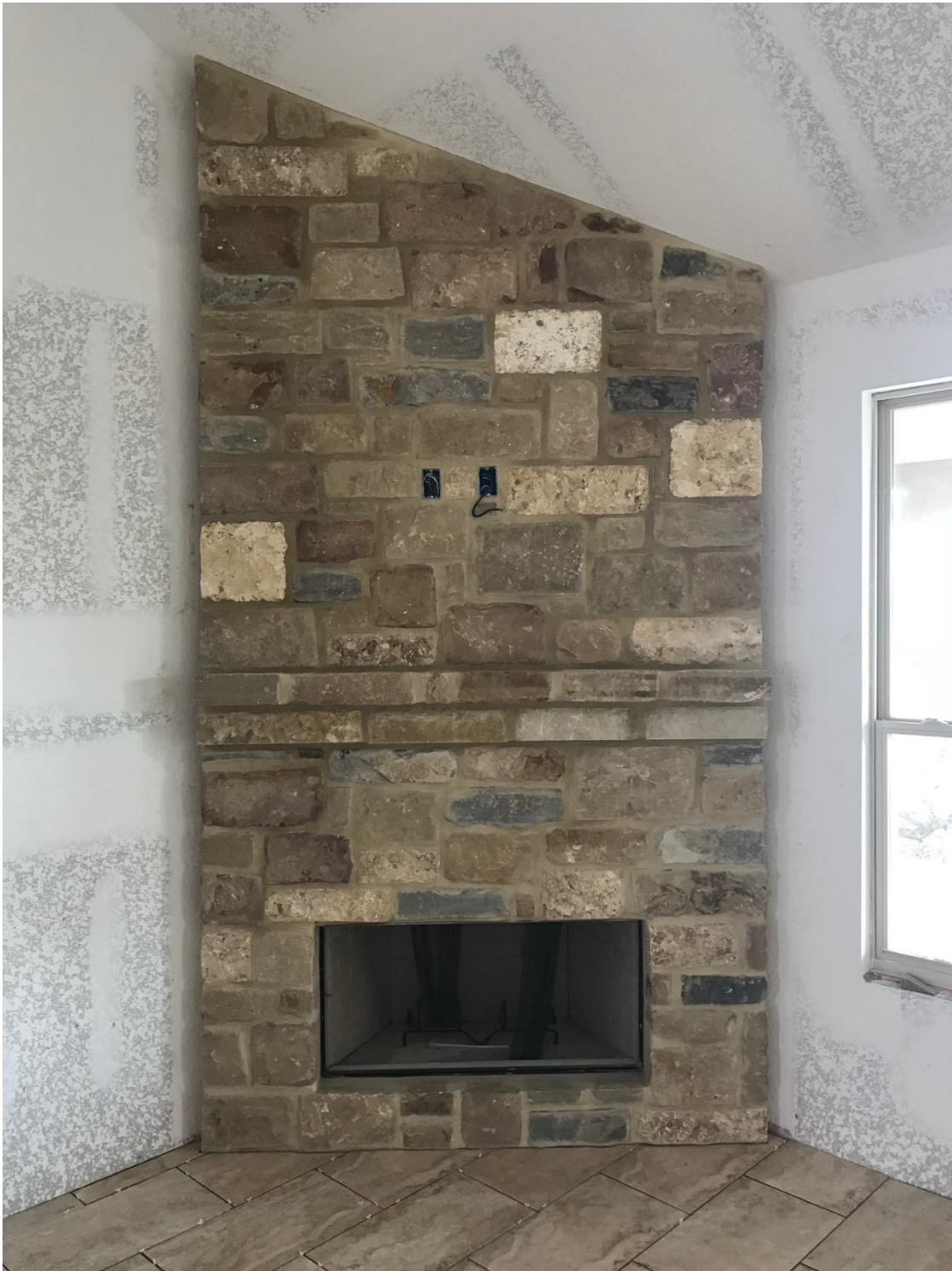
UPGRADE – ROCK TO CEILING AND ROCK MANTLE
